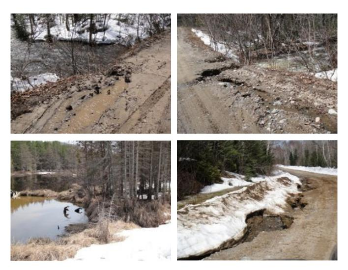
There has been presumptive widening of the road with ill-considered ditching destined merely to relocate and possibly worsen the sedimentation into waterbodies particularly given the use of light sand as road surfacing material. This dusty sand has been scavenged from hillside deposits adjacent to the road and has involved pushing surface material and brush into vernal pools.
